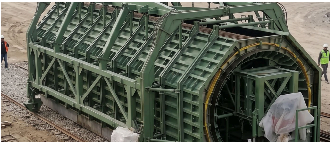
STEEL STRUCTURE FABRICATION
