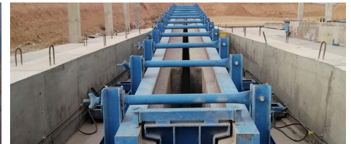
PRECAST MOULD PRODUCTION
